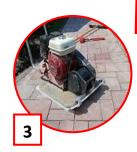
Run plate compactor over surface to compact the sand.
