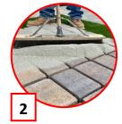
Sweep with a push broom in all directions so joints are filled.
