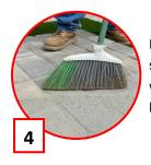
Remove excess sand from surface with a fine-bristle broom.
